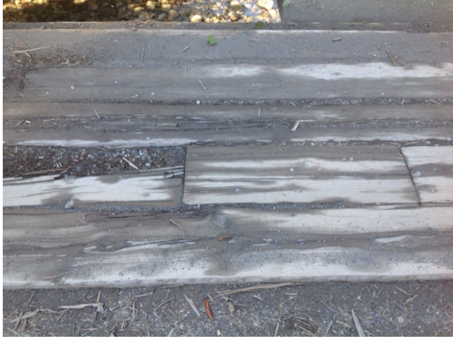
past wear plank replacement
