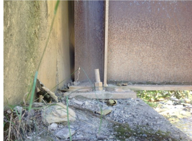
upstream left bearing bolts
