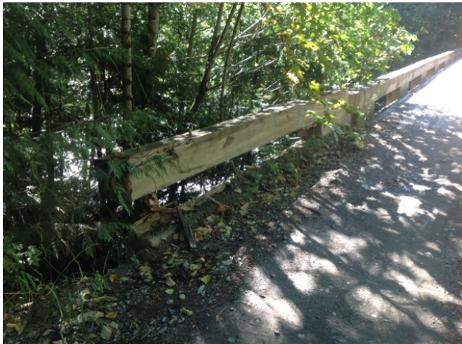
Guard Rail extension onto wing wall on right upstream end
