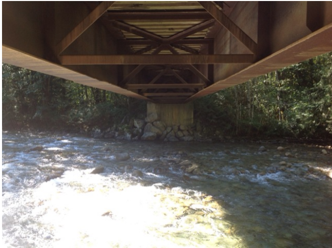
Left Bank Abutment when facing downstream
