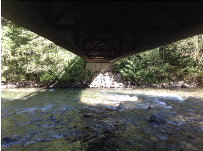
Right Bank Abutment when facing downstream
